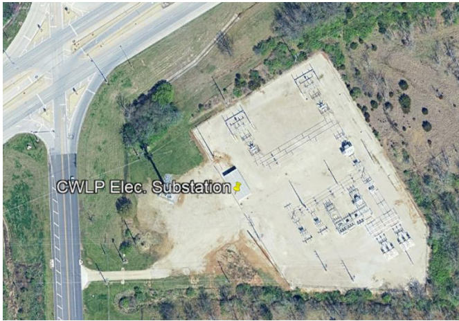
FIGURE 4.10 CWLP SUBSTATION SOUTH OF SPI WITH SPARE CAPACITY
